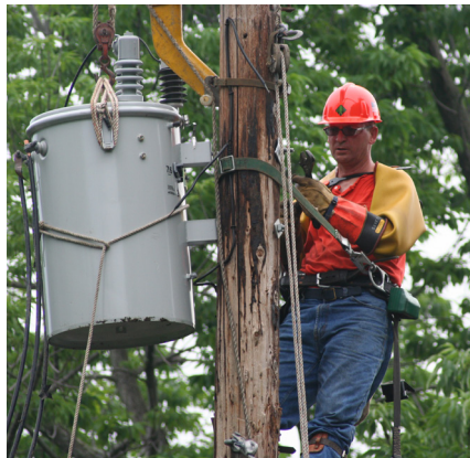
One potential new use for McClellan might be training for electrical linemen, which could build upon the other existing training programs and facilities in this area.
